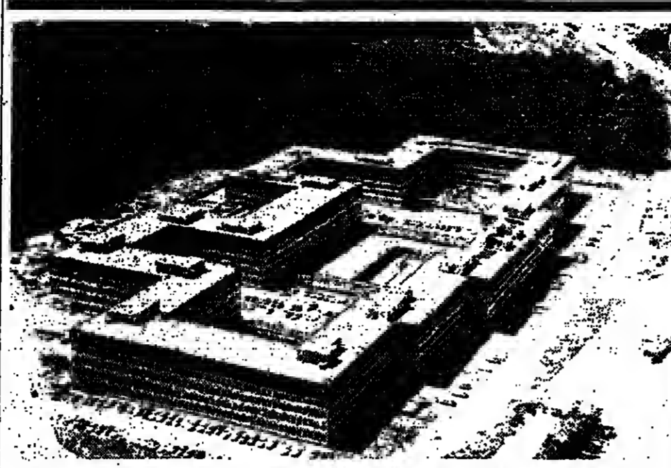
An aerial view of the completed La Boursière office scheme, near Paris.
